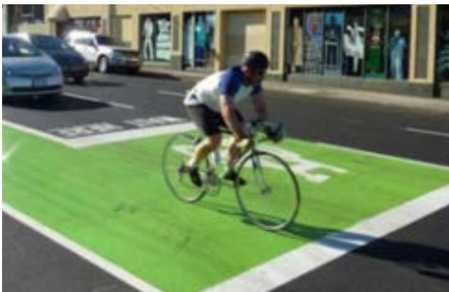
A **bike box** designates an area in front of the vehicular lanes at a signalized intersection. The bike box increases bicyclist visibility by allowing bicyclists to get ahead of queued vehicles during a red signal phase. This treatment can help avoid a “right-hook” conflict between bicyclists and right-turning vehicles.
