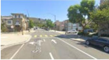
**Curb extensions**, also known as bulb outs, extend the curb line into a roadway at a crossing location. Curb extensions can increase the area available for pedestrians to safely wait before crossing an intersection, reduce crossing distance, and increase pedestrian visibility. Curb extensions can be semi-permanent (striping and delineators) or permanent (sidewalk with curb and gutter), depending upon the characteristics of the roadway.
