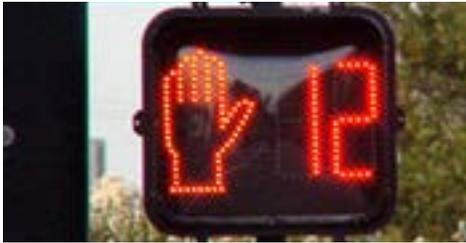
**Pedestrian signal enhancements** improve an intersection’s signal timing, allowing for a more comfortable pedestrian experience. For example, a **lead pedestrian interval (LPI)** is a signal enhancement in which pedestrians receive a green crosswalk signal three to seven seconds before vehicles. This signal timing increases pedestrian visibility and re-emphasizes pedestrians’ right-of-way in a crosswalk.
