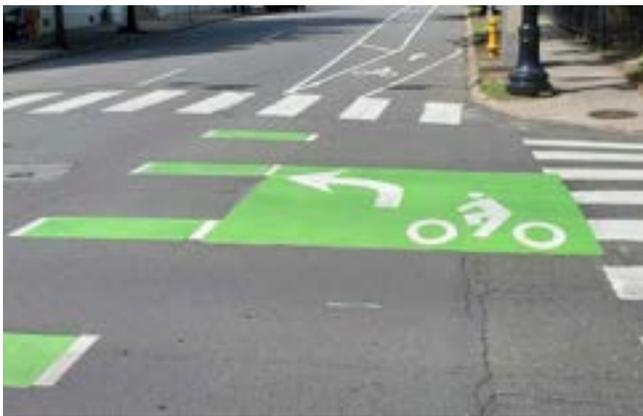
A **two-stage left-turn** box designates an area at a signalized intersection where bicyclists can queue in a right-side bicycle facility to increase comfort when making a left turn. Two-stage left-turn boxes are typically provided when a protected or dedicated intersection is not feasible and the roadway experiences high vehicle volumes or a large number of bicyclists that make left turns.
